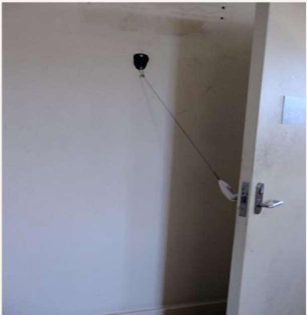
Modified lengthen wiring from fan and electric cable holding door open
