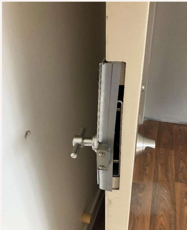
Damaged window with temporary boarding and damaged door handle with internal metal components removed from common area door in accommodation compound
