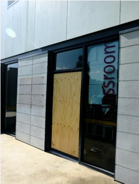
Damaged Doors – board replacing door and missing handle
